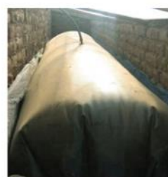
Tube Digester Altiplan of Bolivia
